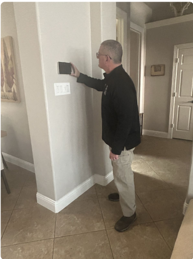
A Stonebriar inspection: operating a thermostat during an inspection to confirm the system responds in heating and cooling modes.
