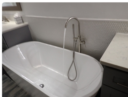
Stonebriar field photo: a freestanding tub with a hand shower. Delivered temperature at the fixture is what matters for scald protection.
