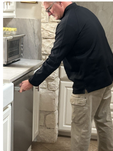
A Stonebriar inspection: operating a dishwasher during an inspection. After installation or service, watch a complete cycle and recheck the floor and toe-kick.
