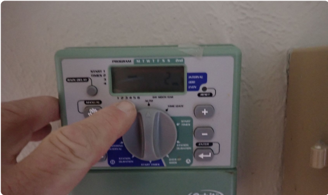
Stonebriar field photo: an irrigation controller. Photograph the program before seasonal changes so a provider can restore it.
