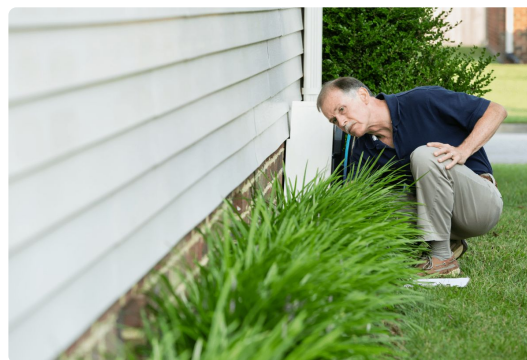
Stonebriar field photo: measuring along the foundation perimeter. Repeatable measurements from the same reference points make later comparisons meaningful.
