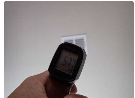
Stonebriar field photo: a non-contact thermometer reading at a supply register. Spot readings describe one moment; they do not diagnose the equipment.
