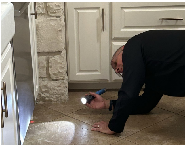
A Stonebriar inspection: checking the floor and cabinet base beside a sink with a flashlight. Monthly cabinet checks catch slow leaks before cabinets swell.
