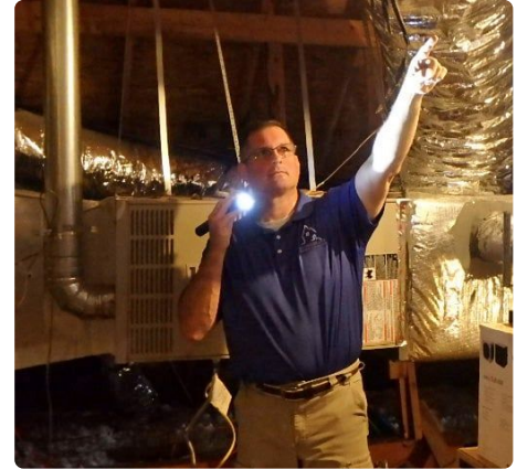
An inspector in an attic beside HVAC equipment and ducts, observing from a service platform.
