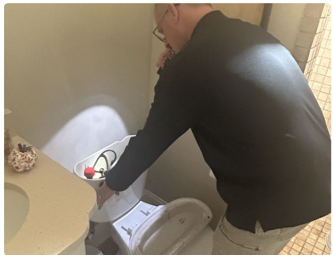
Checking a toilet for movement, leaks at the base, and continued running after the cycle.
